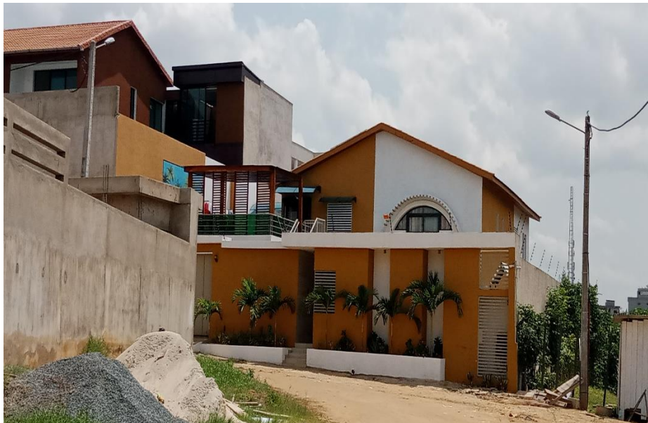
Figure 6. Good Standing Housing built by the INTERBAT Company in Cocody. Source: Deki shooting , April 2024.
