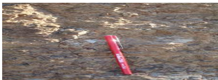
Figure 6b. Outcrop showing soil characteristics with deep cracking and shale fragments (author own research, 2014).
