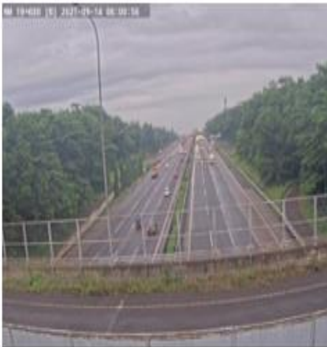
Figure 4. Research location, Jagorawi toll road KM 19+600.
